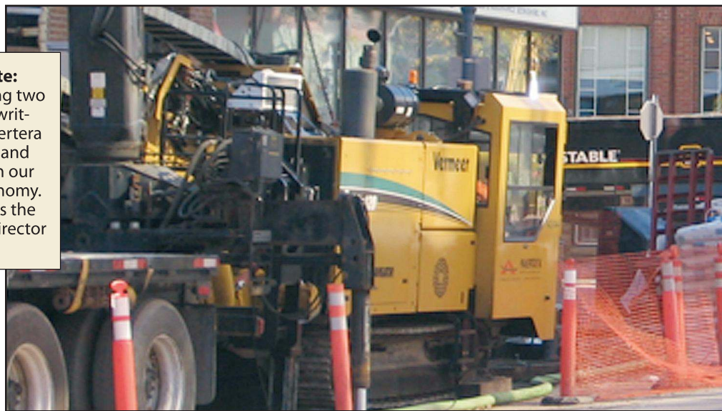
Sewer being upgraded in downtown Moncton
